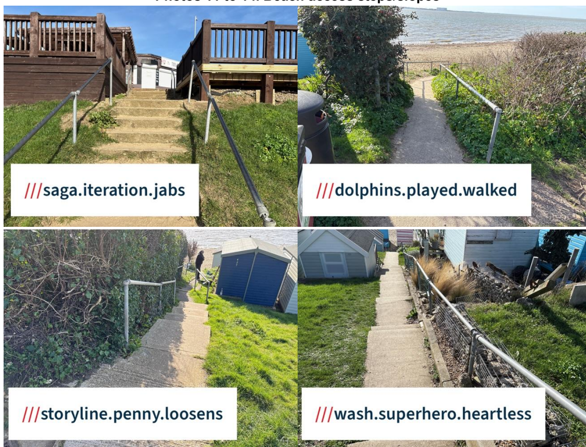
Photos 11 to 14. Beach access steps/slopes
